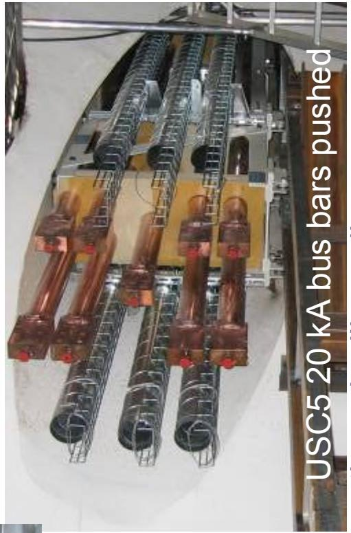
USC5 20 kA bus bars pushed through pillar wall
