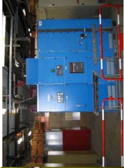
20 kA power converter tested
